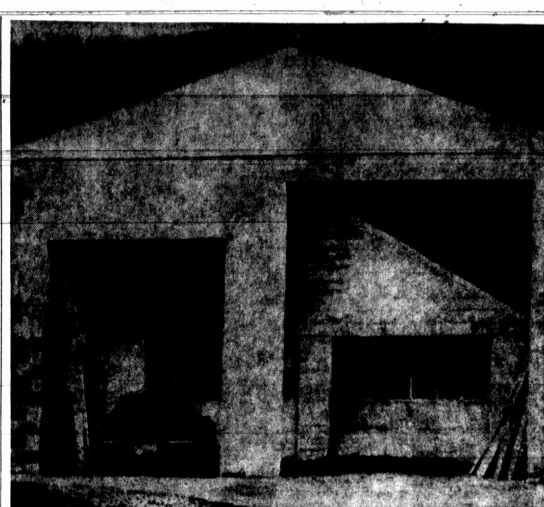
FOR THE MAN WHO HAS EVERYTHING—This is an ideal Christmas gift for the motorist who has everything: A garage to keep his garage in. Actually, this Reading, Pa., construction project calls for the smaller garage to be dismantled after the larger building is completed. In the meantime, the owner still can keep his car under roof. (AP WIREPHOTO)
