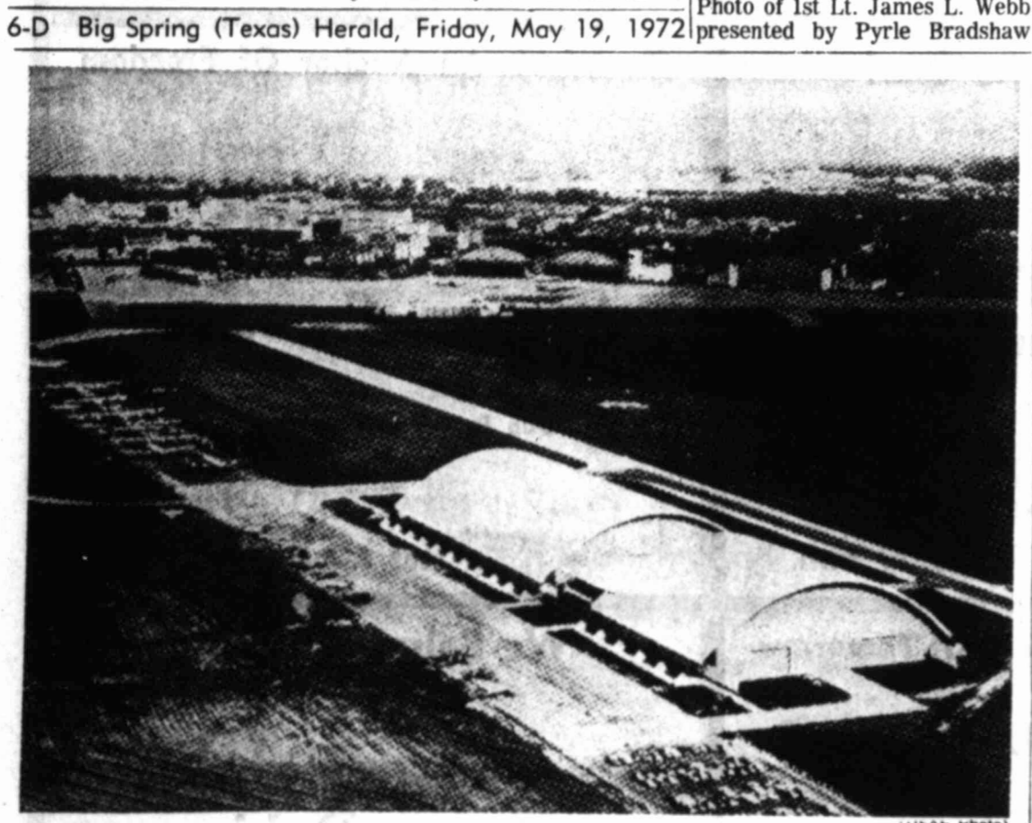
THE AIR FORCE MUSEUM , in a new arch-type structure comparable in design to many early aviation hangars, provides a dramatic setting for 80 historic aircraft to be displayed. Located parallel to the runway at Wright Field, Dayton, Ohio, the new building is 800 feet long. Interestingly, the building's 240-foot width is twice the distance of the Wright's first flight in 1903.
