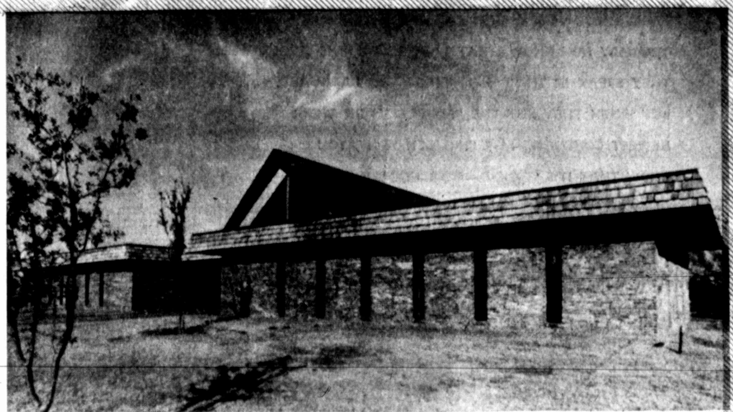
LONG-TIME DREAM MATERIALIZES AT BIG SPRING STATE HOSPITAL Tollett All-Faith Chapel made available to worshippers at facility here
