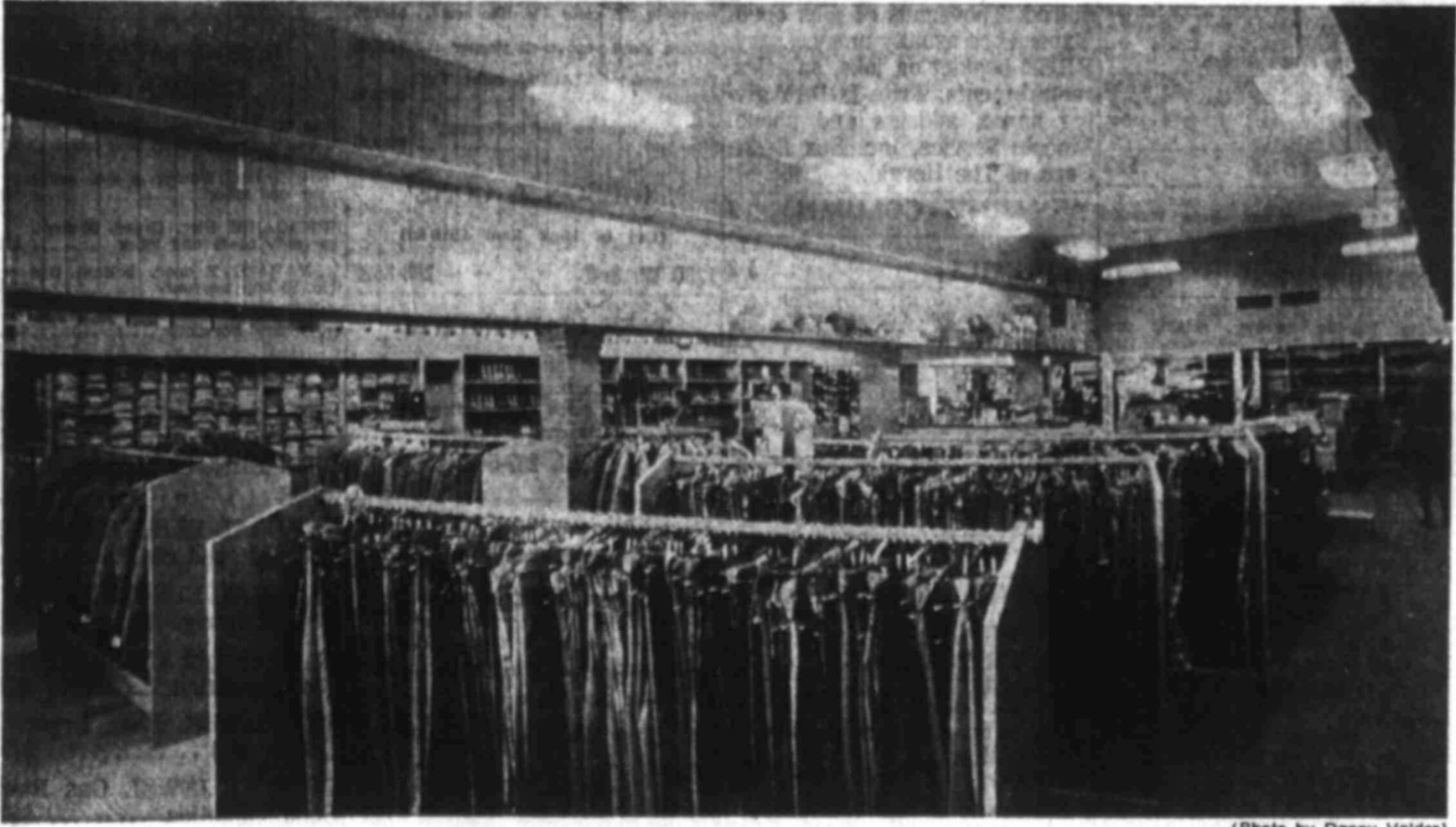
WESTERN WEAR SHOP REMODELS STORE ... increased inventory, more display space
