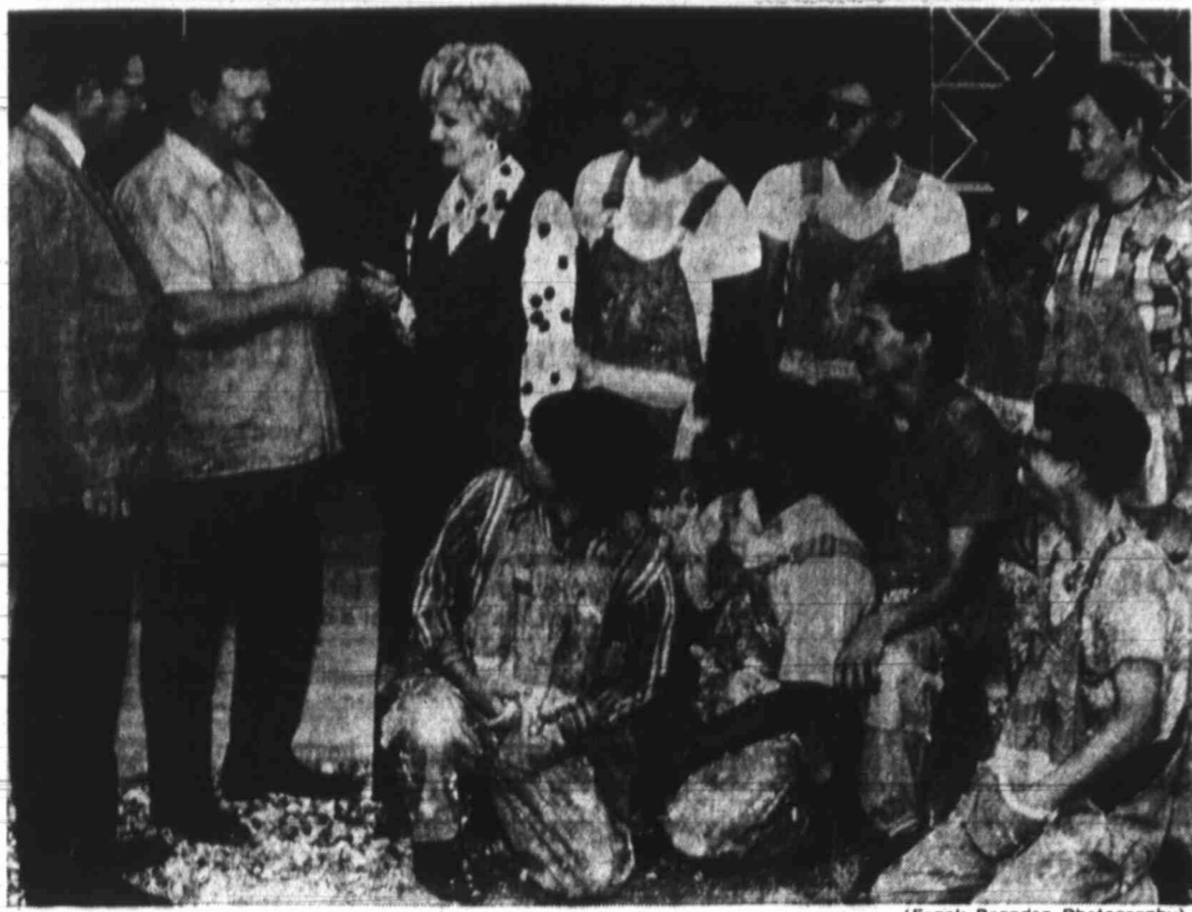
HERE ARE THE KEYS — Jerry Woods, instructor in vocational building trades at Big Spring High School, hands over the keys of a new house to Mrs. R. B. Hall while John Bagnall, head of the vocational division, and some of the class members watch. Students in the class built the house on Moss Creek road as a project under supervision of Woods. Others, standing, are Benito Rubio, Pascual Porras, Ferney Hernandez and Gary Dunlap; kneeling, Rick Monteleone, Joe Chavez, Jesse Olague and Kenneth Evans.
