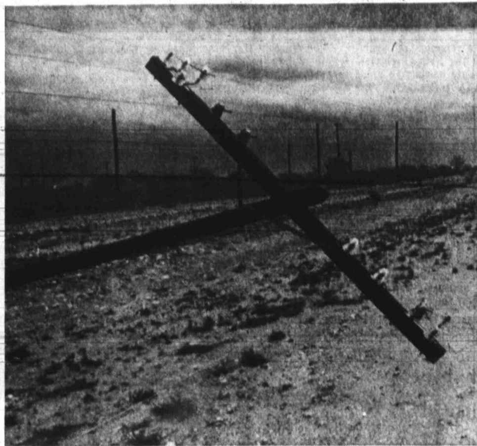
WINDS DOWN UTILITY POLE
