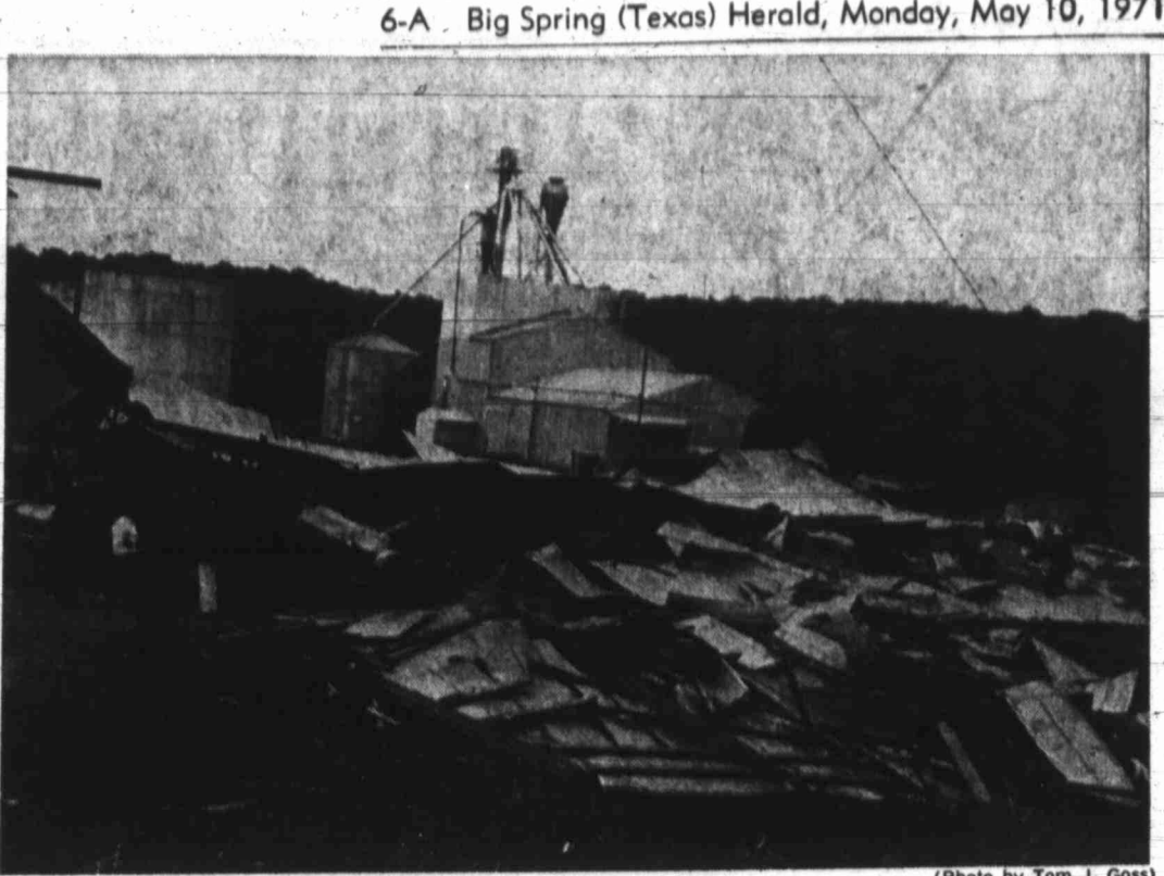
WIND DAMAGE — This building used to store cotton seed hulls was flattened and scattered over the west end of Front Street by high winds Saturday night in Colorado City.
