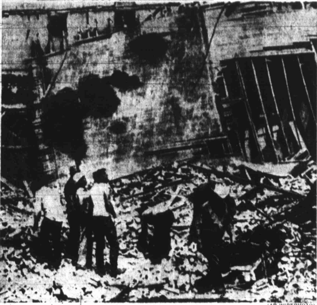
DEATH FOR THREE — Three construction workers were crushed to death Wednesday when one wall of this four-story building on Oklahoma City's main street collapsed. The men were helping demolish the building. Their bodies were recovered Wednesday night.
