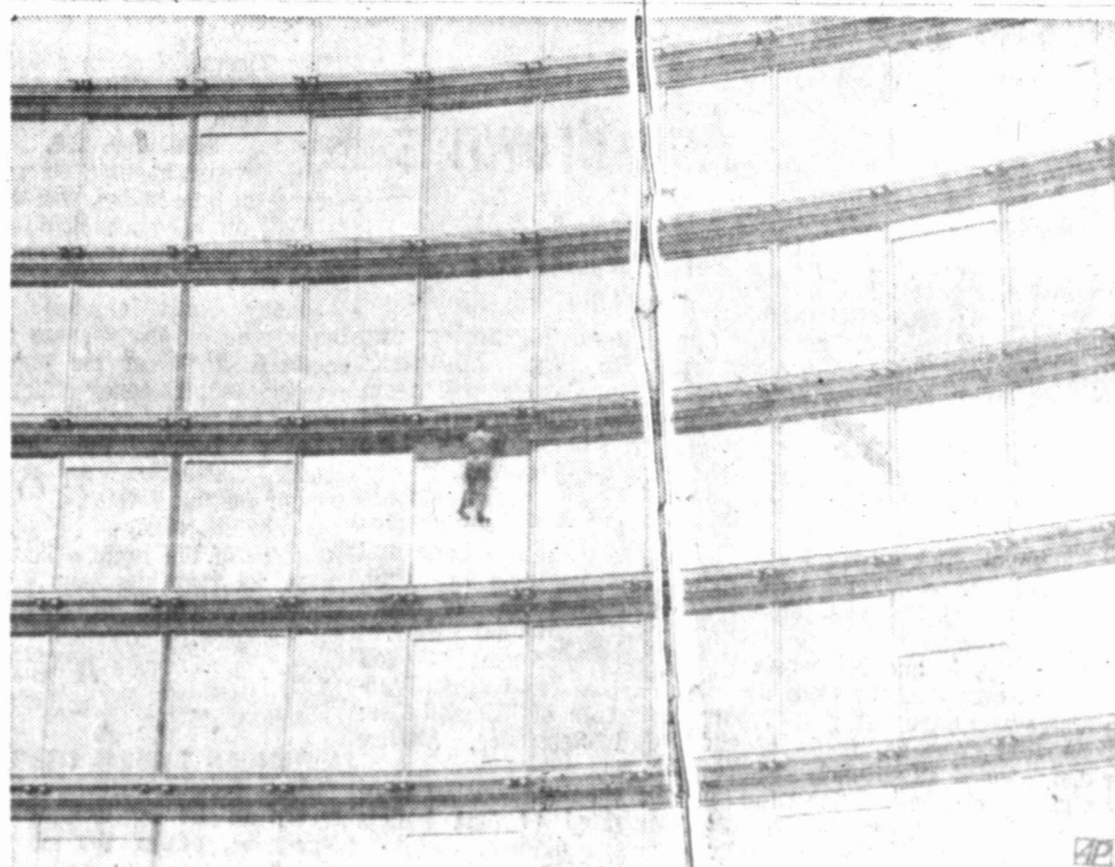
OVER AND OVER AGAIN — Taking care of all the windows of the Berlaymont building is a constant task for this window cleaner in Brussels, Belgium. Structure houses the ECC committee that meets and prepares legislation for Common Market countries.
