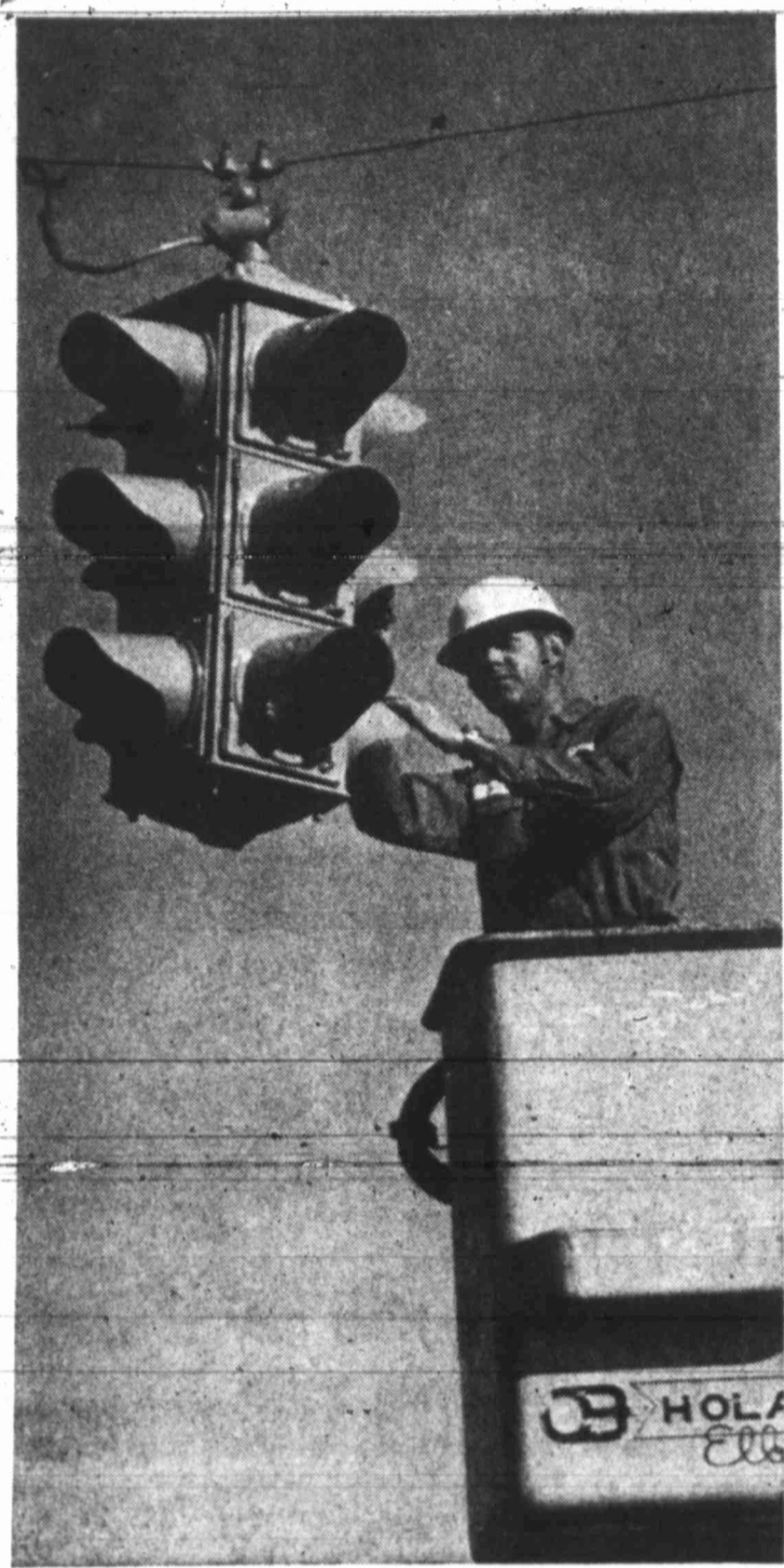
TEDIOUS WORK Jim Parrish paints signal
