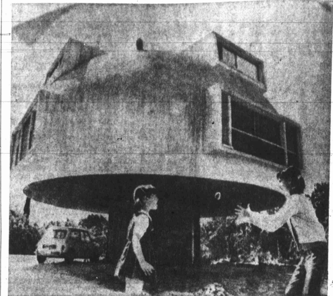
MUSHROOM HOUSE — A "mushroom house" in Rehovot, Israel, home of the Ravid family, is an example of a newly-developed way of home-building being tried out in Israel. The house, which is relatively inexpensive to build in addition to being a conversation piece, "sprouts" from a central pillar, which also serves as an entrance. The net result is a combination cellar-porch, which must be attractive to the youngsters on rainy days, and a cool place to relax when the sun beats down.
