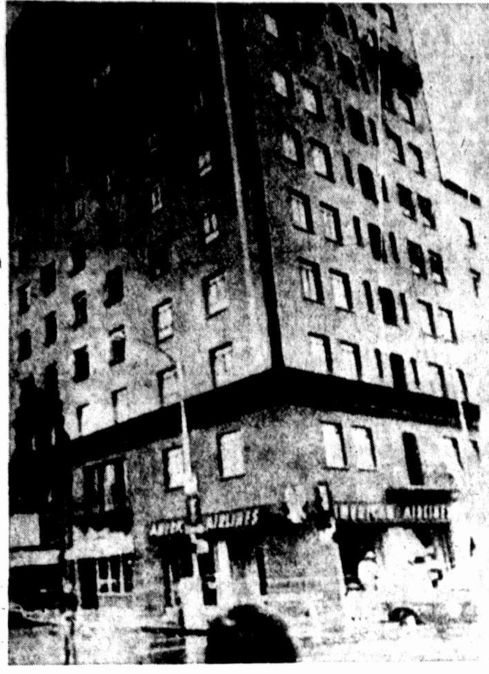
WHERE PEOPLE TRAPPED IN FLAMING HOTEL—At least 28 persons were killed Sunday when fire struck the Pioneer International Hotel in Tucson, Ariz. The 12-story hotel shown later Sunday. At right, bed clothing is tied to windows
