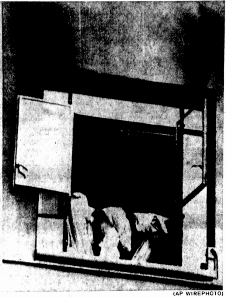
where residents attempted to lower themselves from lower-level windows. Fire ladders could reach no higher than the eighth floor, and many residents jumped to their deaths.
