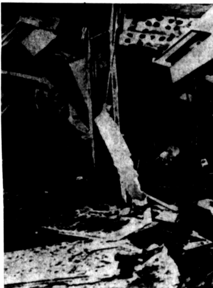
UNIVERSITY OF OREGON — Investigators searched for clues after an apparent bombing damaged the ground floor of the nine-story Prince Lucian Campbell Hall on the U of O campus. There were a few people in the building at the time of the blast but no one was hurt.
