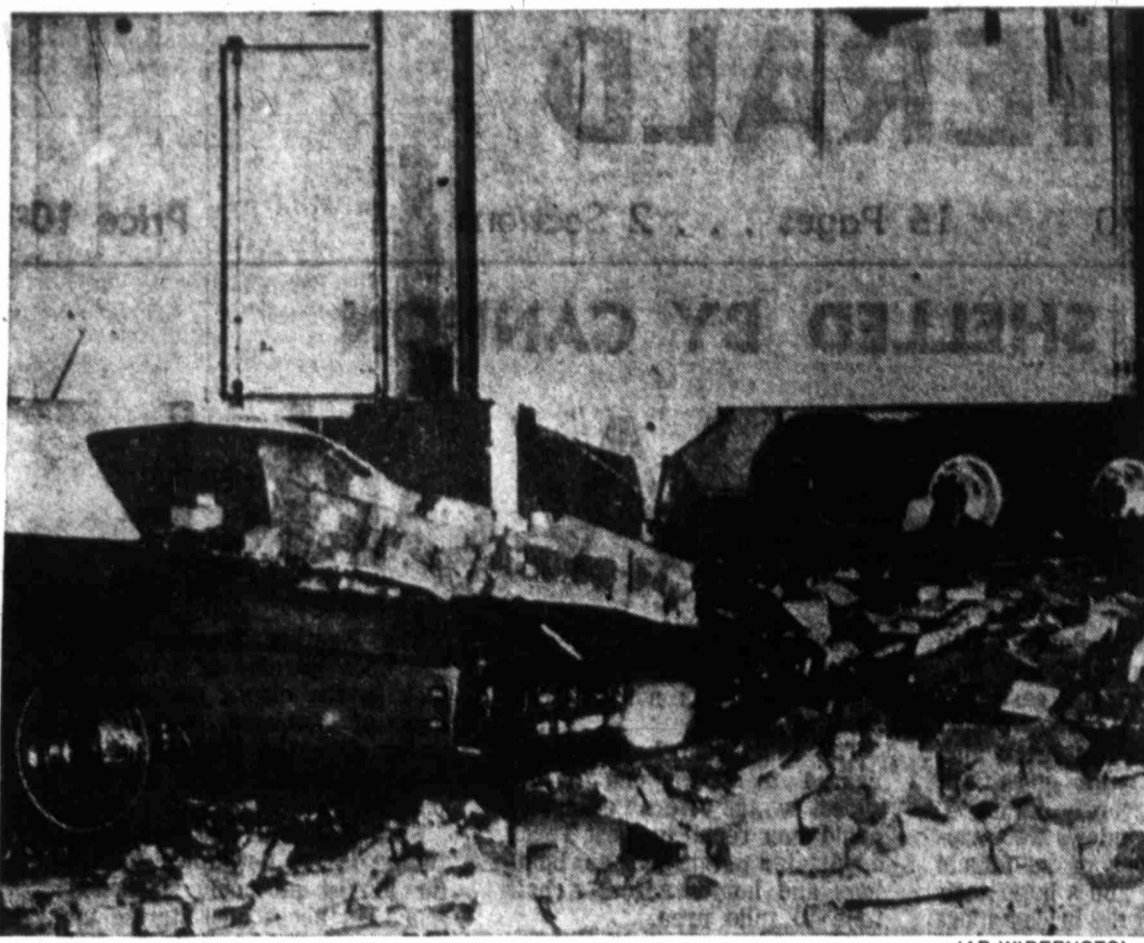
DAMAGED AVALANCHE-JOURNAL — The Lubbock Avalanche-Journal is one of the many buildings hit by two tornadoes that ripped through the city shortly before 11 p.m. Monday. The tornado that hit the downtown area killed more than 20 people and hundreds more were injured.
