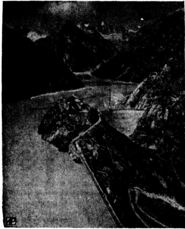
HIGH SIGHT — The dam at the Grimsel Pass forms a lock across the valley to store water for electric power in the Bernese Oberland region of Switzerland.
