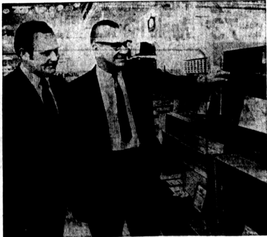
LOOKING OVER NEW AIR CONDITIONERS ... G. B. McElroy and Ernie Pannell (right)
