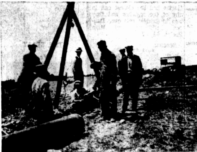
HAND LABOR —Digging in the hard rock of Section 17 was all done by hand labor back in 1929, and the wooden A frame was the only mechanical help the crews had to lay this 12-inch pipe, which came in six-foot lengths.
