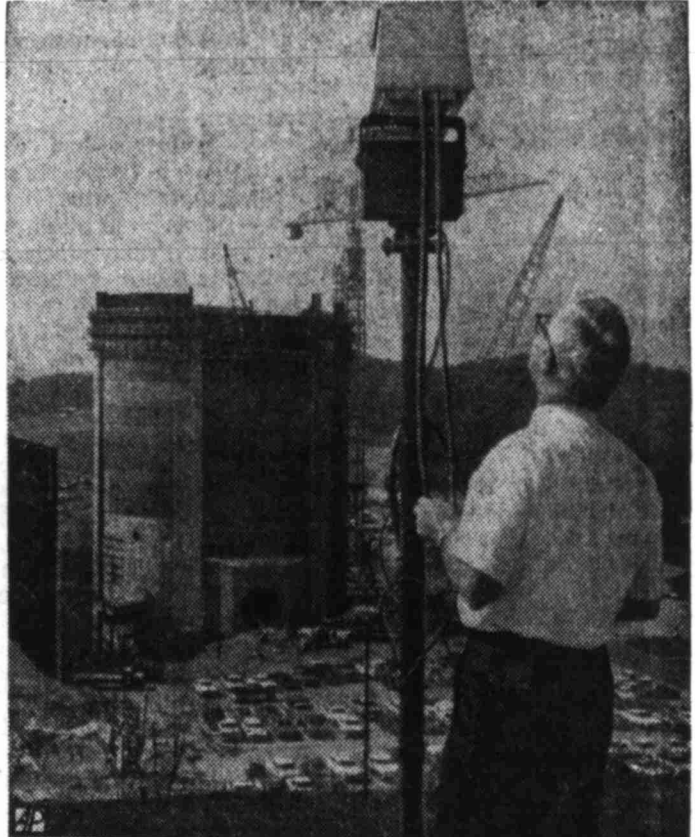
MODERN EYE — Passersby are given assist by construction company which set up a TV view of the giant nuclear power plant being built near Greenville, S. C.
