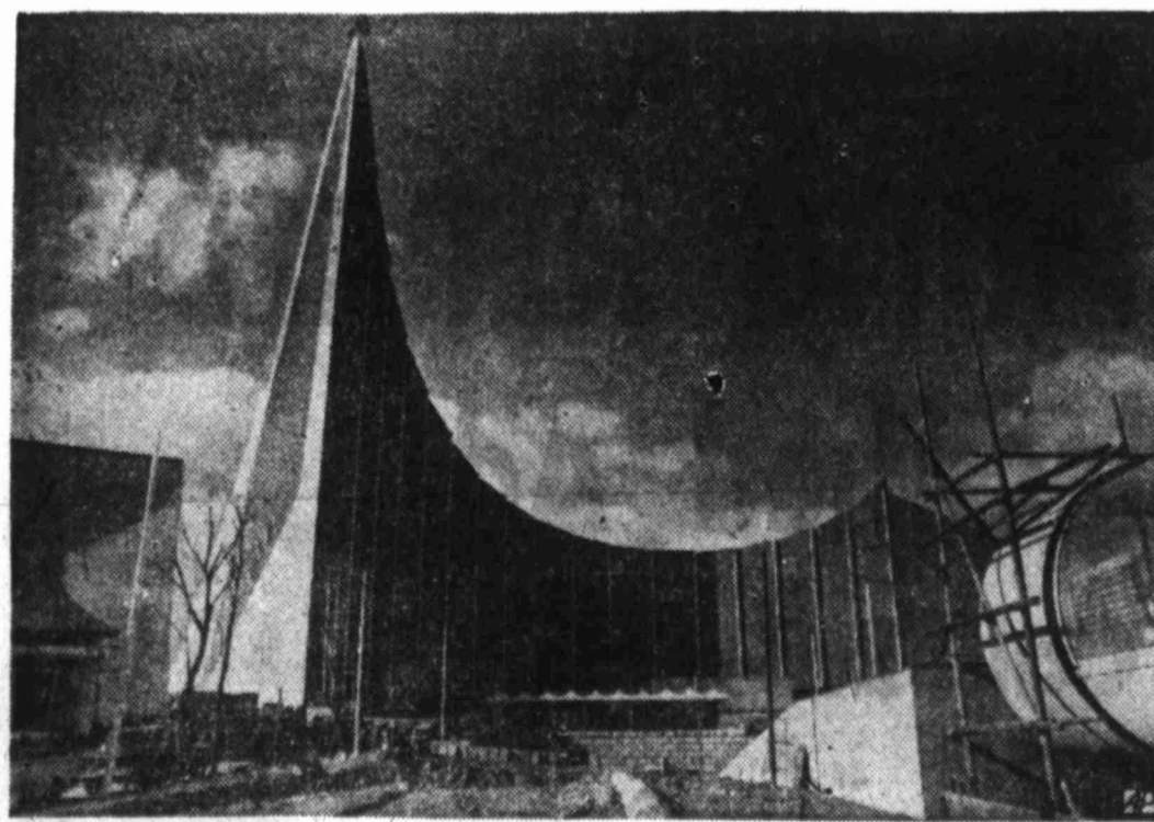
RISING INTO THE SKY — The Soviet pavilion nears completion at the Expo 70 site near Osaka, Japan. Hammer and sickle-topped structure is the tallest on the site.
