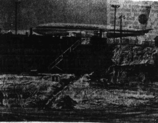
BUSINESS AS USUAL - A jetliner prepares to leave during excavation for the below-ground floor of a new passenger terminal at Kennedy Airport in New York. A sheet piling cofferdam holds back the waters of Jamaica Bay 22 feet below ground level.
