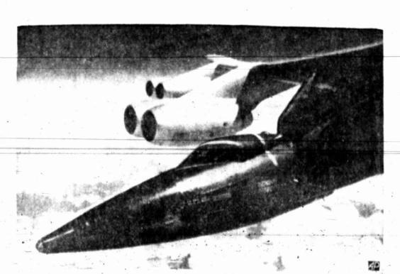
UNDER THE WING - An X-15 rocket plane is carried under wing of a B-52 bomber before being air launched. After 199 flights, the X-15 program was concluded late last year. The number one plane will enter the Smithsonian Institution in late May.
