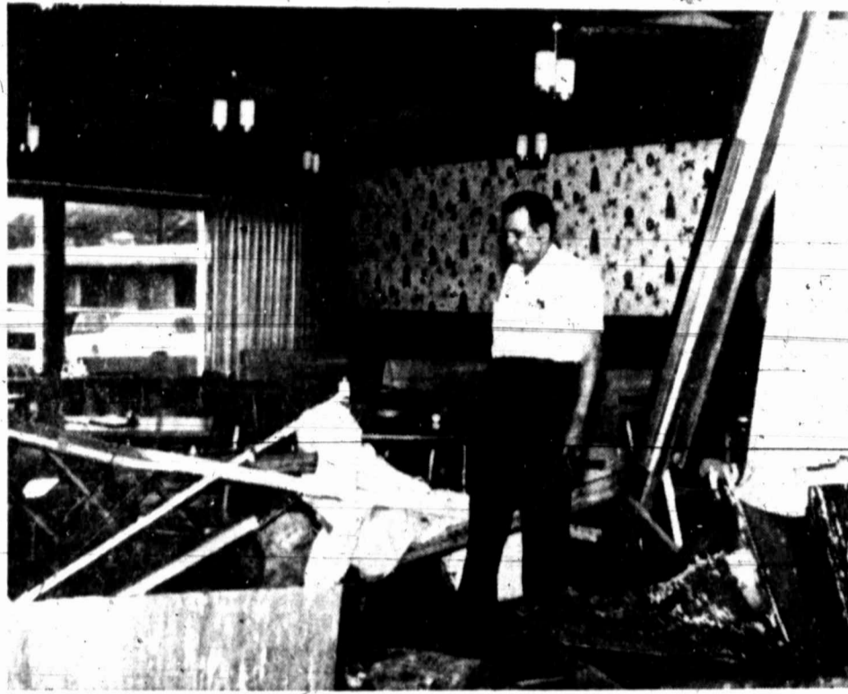
PICKUP TRUCK CAUSED THIS DAMAGE M. C. Bodine, proprietor, surveys damage to Ponderosa Restaurant
