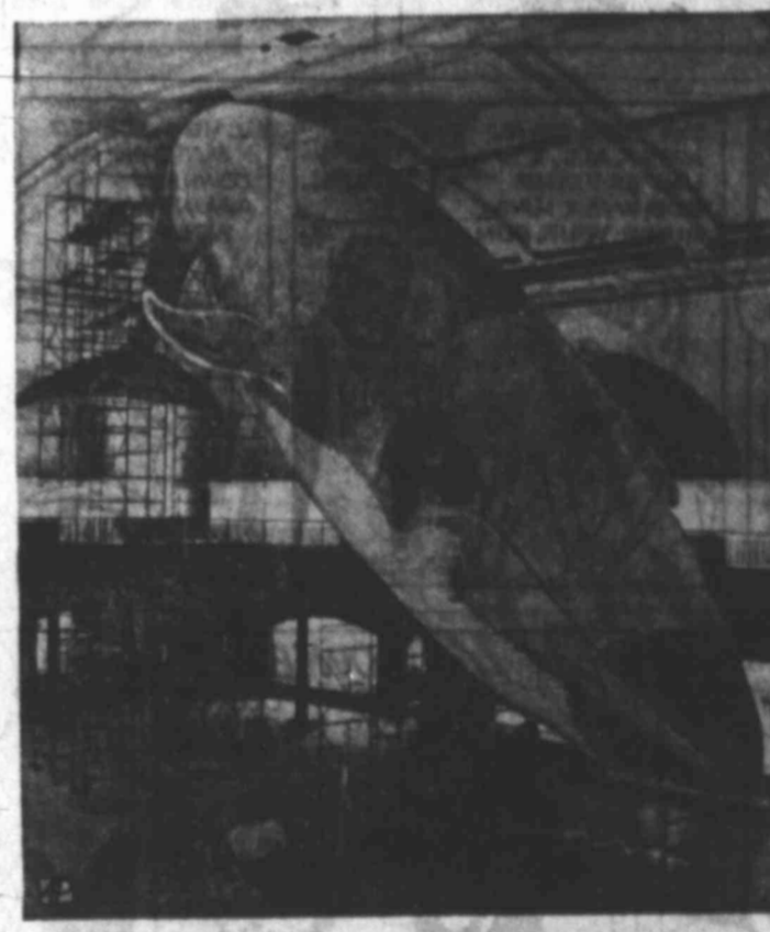
NEW 'STAR' — Here's the American Museum of Natural History's new giant Blue Whale made of steel, plastics and fiberglass. It replaces an old plaster model.
