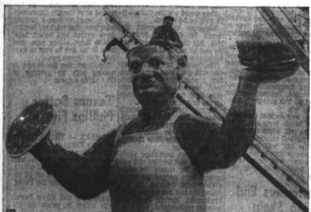
AT THE 'CONTROLS' — Enterprising photographer pictured the scene as Henry Severson was installing the electrical "brains" in a 30-foot high sign in Portland, Ore.
