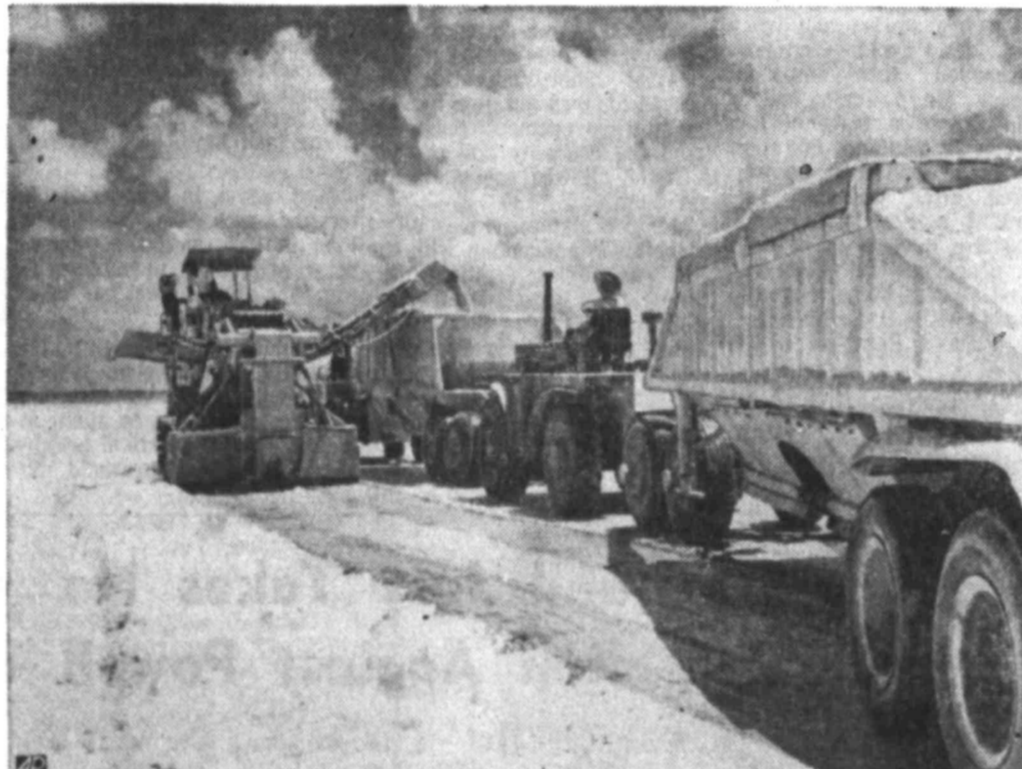
SCRAPING UP SALT — A harvester removes salt from crystalizers at the Diamond Crystal solar plant in the Bahamas. Trailers carry the salt to process plant where it is washed and dried for shipment to manufacturers and agencies in the United States.
