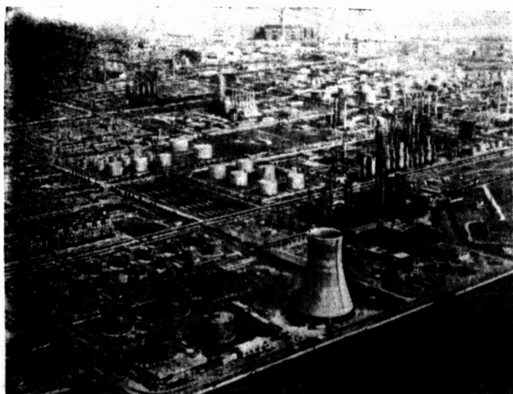
MODERN TOUCH IN ROMANIA — One of the biggest and most modern oil refineries in Europe is at Brazi in Romania. Romania's complete crude oil extraction is processed here. The catalytic cracking installation has over one million ton capacity.
