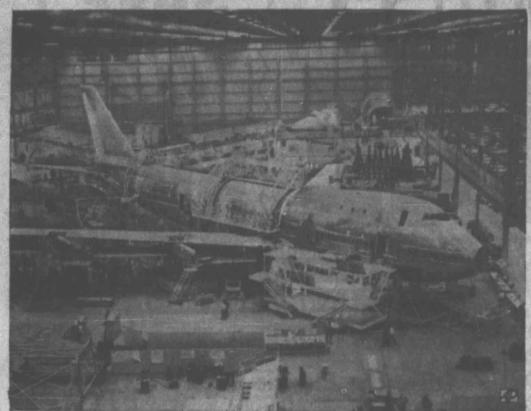
BIG JOB IN PROGRESS — The Boeing 747, among the world's largest commercial jetliners, takes shape at the company's plant in Everett, Washington, after main section of the wing, fuselage and tall were joined, it will seat over 350 persons.
