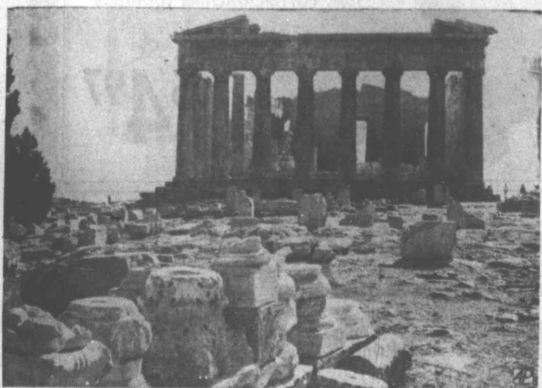
TEMPLE IN JEOPARDY — The famed Parthenon in Athens, Greece, is threatened with collapse. Water seepage, tourists, air pollution and jet vibrations are being blamed. A UNESCO mission from Paris is en route to ascertain means of preservation.
