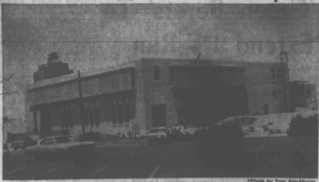
NEW FACILITY IS FAR AHEAD OF SCHEDULE Contractor to wind up work on Post Office by mid-November
