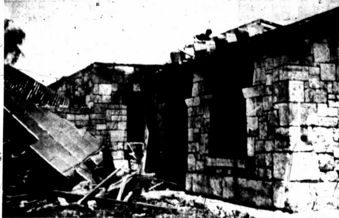
VANDAL-RUINED STRUCTURE IN STATE PARK BEING RESTORED. Main building is to resume its original attractiveness.
