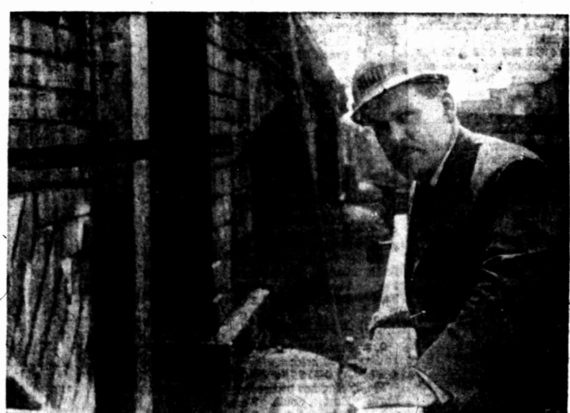
SHOULDERS TALL TASK — Henry Colley, 40, is engineer in charge of dismantling stone by stone the London Bridge. All the stones are numbered so that bridge can be rebuilt at Lake Havasu City, Arizona. A U.S. oil corporation bought bridge.
