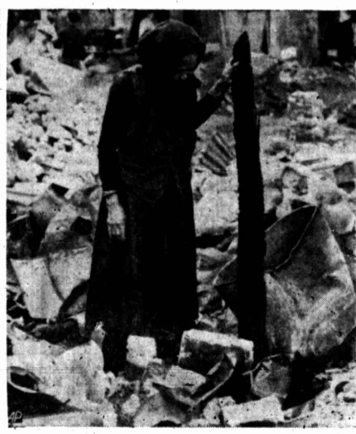
LITTLE LEFT — An old woman sifts through the rubble of what once was her brick and tin-roofed domicile in the war-devastated city of Hue in South Vietnam.
