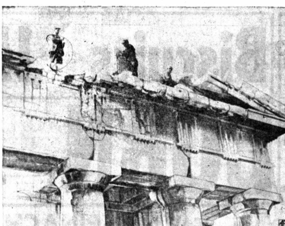
PROPS NEED SUPPORT — Workmen examine the masonry of the marble propylae columns leading to the temple of the Parthenon on the Acropolis in Athens. The 2,500-year-old columns have been weakened by time and vibrations from low-flying aircraft.
