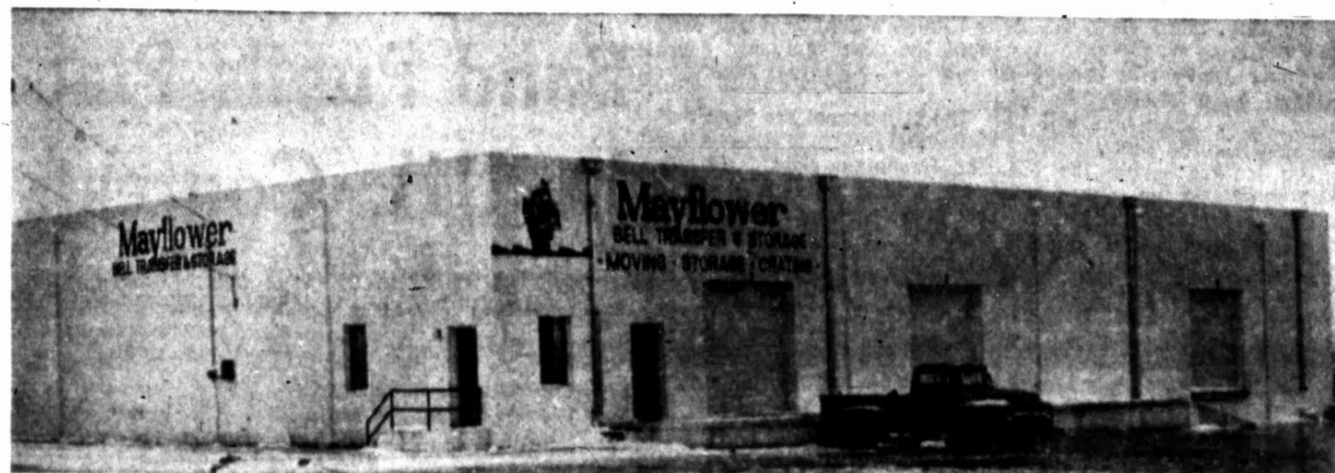
NEW MAYFLOWER WAREHOUSE AND OFFICE
