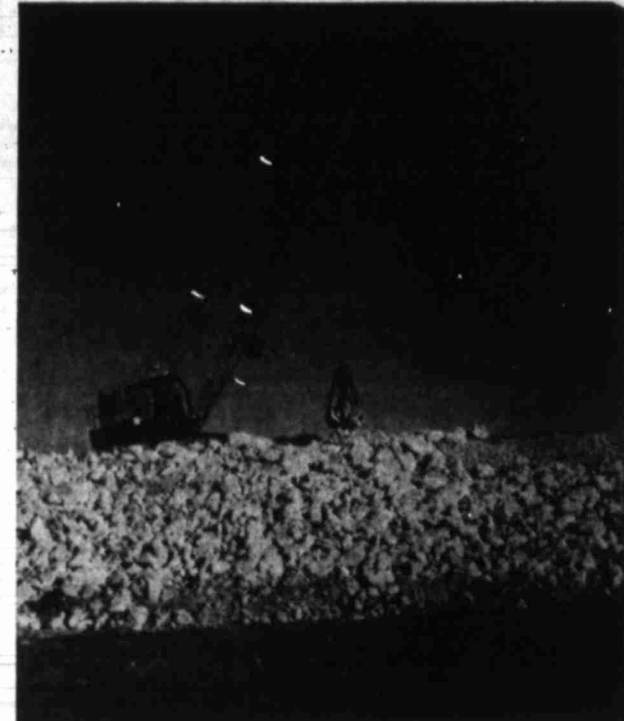
Rip rap put on dam
