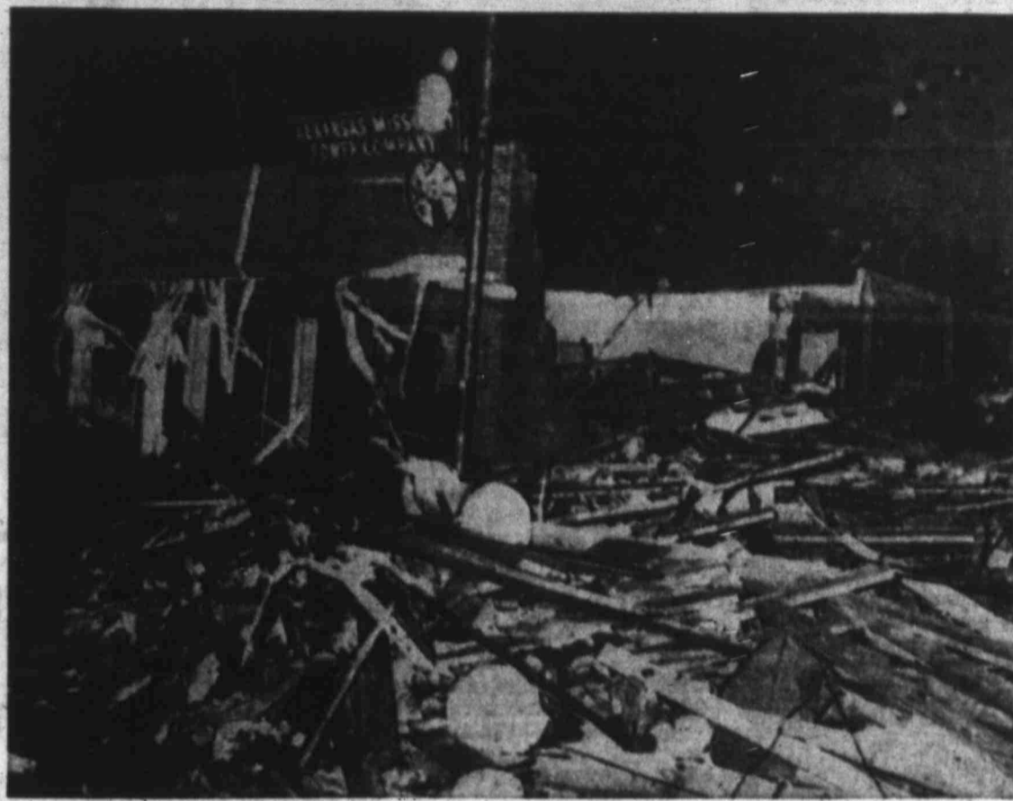
Demolished Utility Office
