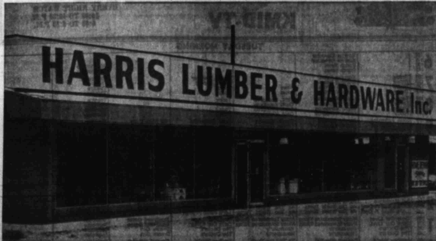
HEADQUARTERS FOR LUMBER AND HARDWARE NEEDS Offers dozens of ways to decorate any room of all homes
