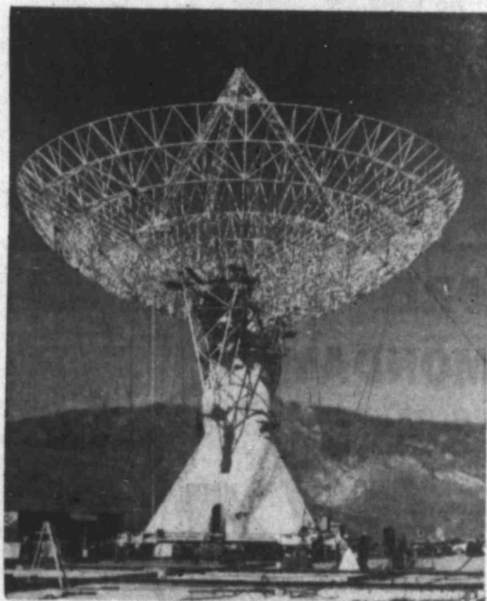
THE BIG TOPPER —The 130-foot dish antenna dominates the California Institute of Technology's huge new radio telescope installation in the Owens Valley.
