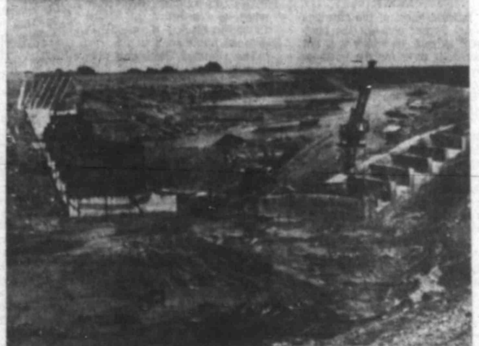
Looking West From Stilling Basin
