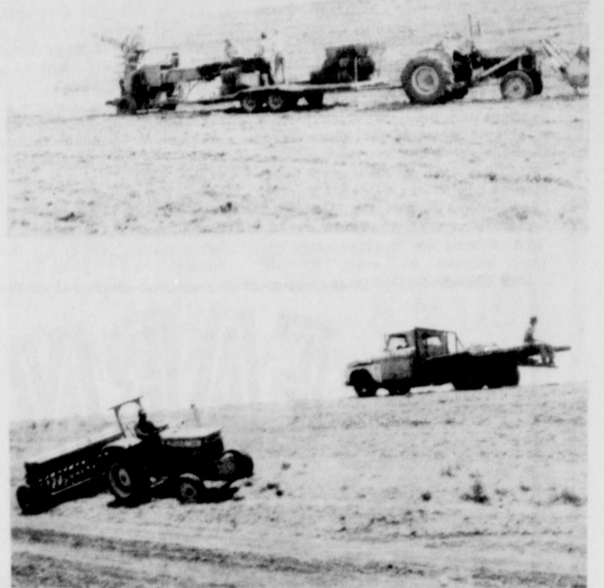
RESEEDING DAM... Employees of the Bachmayer Company, which has been contracted to reseed grass on the Bovina Dam, in the top photo, are shown blowing prairie hay mulch on the dam as part of the reseeding operation. Eleven different kinds of grass have been planted on the Bovina Dam as part of the reseeding operation to protect it from erosion. (SCS Photos)
