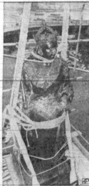
ON THE MOVE —Bronze statue of Queen Victoria, perched for 71 years at north end of Blackfriars Bridge in London, is moved to a new site in the course of progress.
