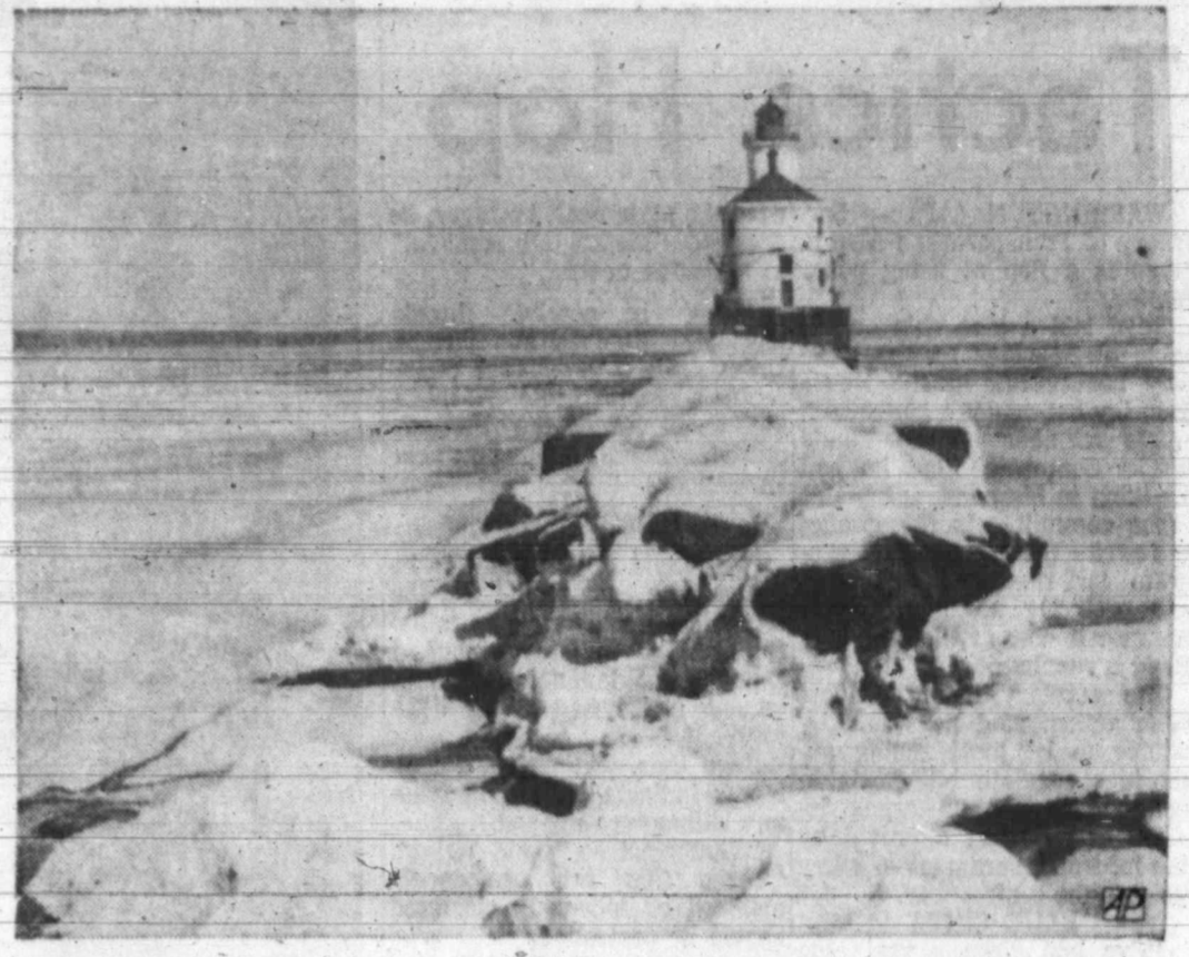
WAITING FOR A THAW — It may be spring elsewhere but winter's grip is fast on the Superior, Wis., harbor entry breakwater. Lighthouse was left an island by winter storms and it will have to be restored for the Lake Superior navigation season.
