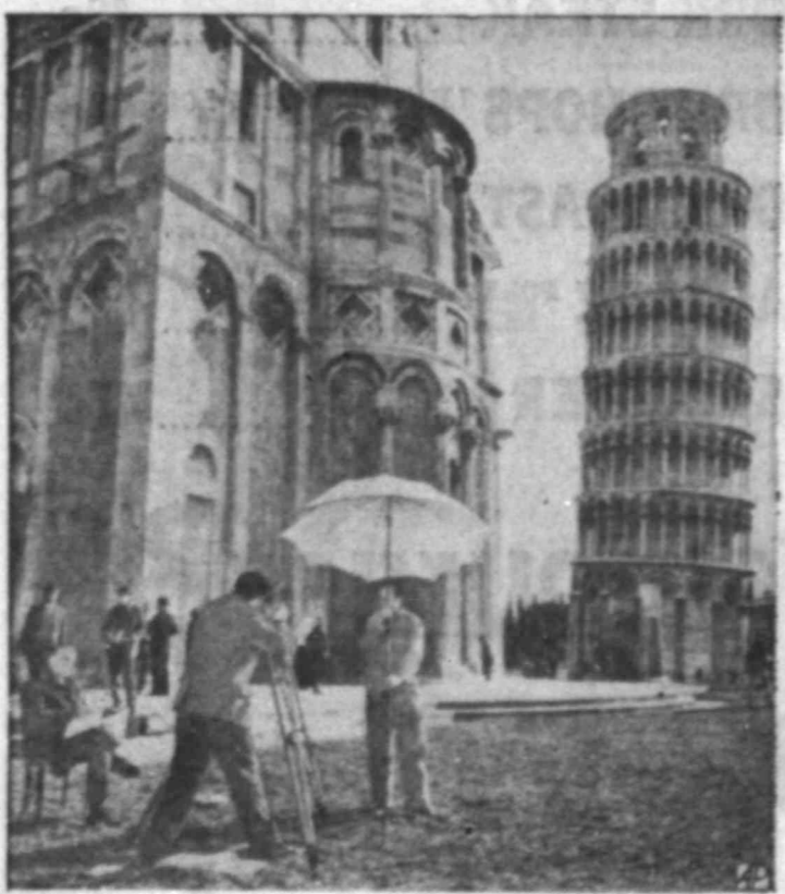
LEAN TASK —Technicians measure tilt of the Leaning Tower of Pisa in one of periodic controls of the 13th Century Italian landmark which stands 179 feet.
