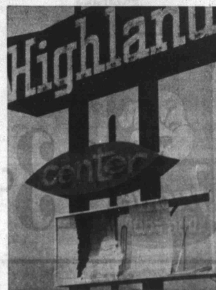
SIGNBOARD DISPLAY AREA SHATTERED Will have to be repaired
