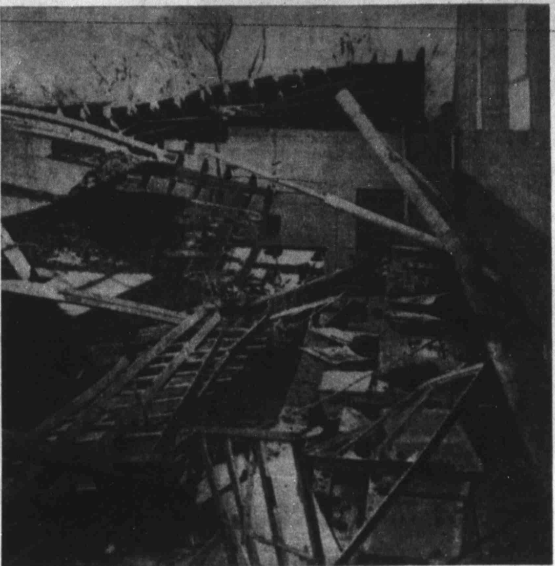
The Roof Fell In
