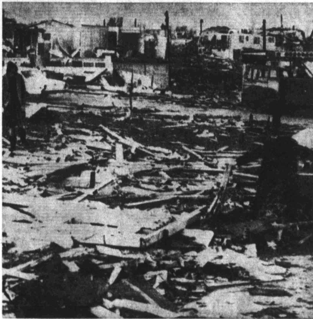
Twister Destruction Near St. Louis
