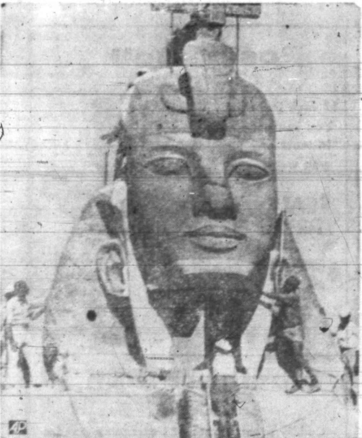
SET IN PLACE —One of the heads of the four rock-hewn colossi of Ramses II is hoisted into position on the new site of Abu Simbel temple at the Aswan Dam.
