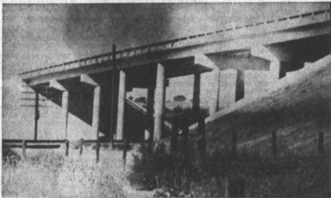
NORTH LEG OF FM 700 SOON TO BE PUT INTO SERVICE Overpass at T&P tracks major structure on newest county highway
