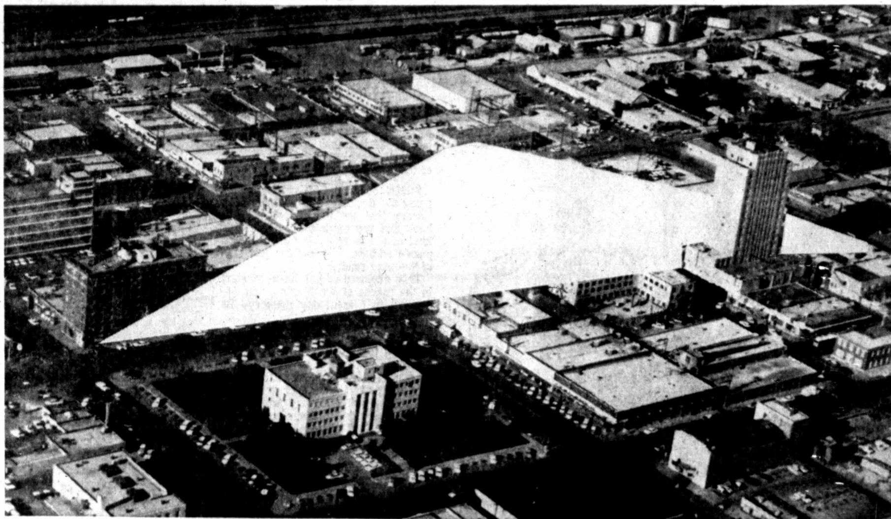
WHITE INSET SHOWS APPROXIMATE SIZE OF NEW COLORADO RIVER DAM Structure rises 143 feet from river bed, plus another 30 feet from core trench
