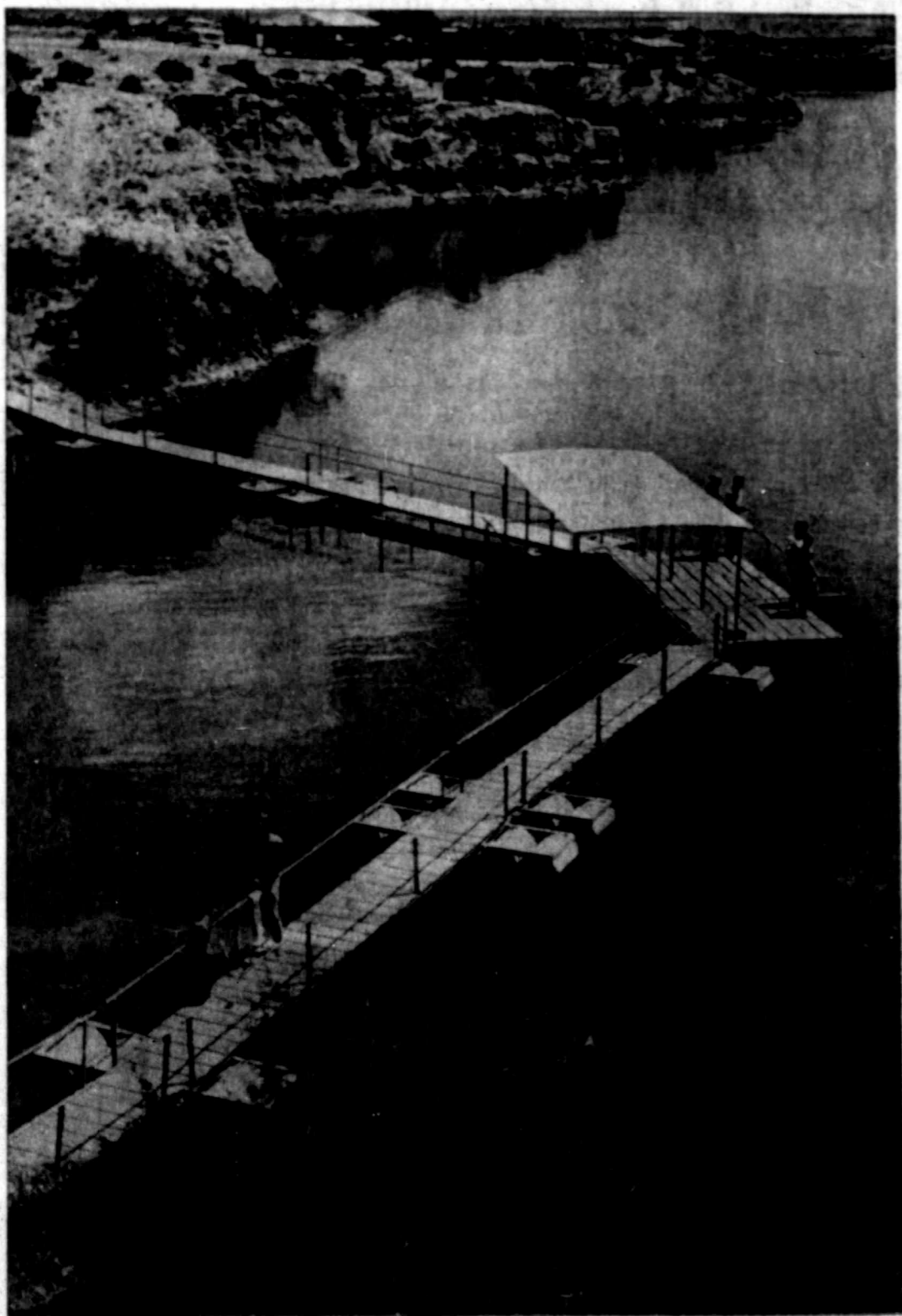
PIER PROVIDES PLACE IN THE SUN
