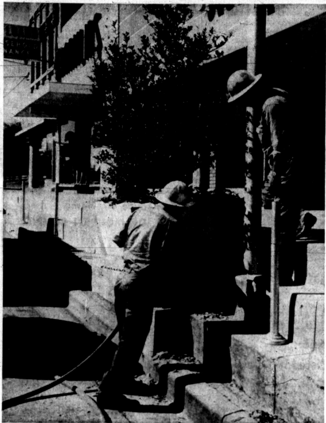
Work Gets Started
