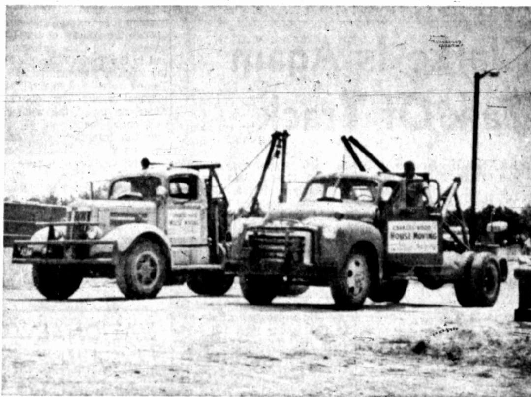
READY TO MOVE YOUR HOUSE Charles Hood's trucks can do the job efficiently, quickly
