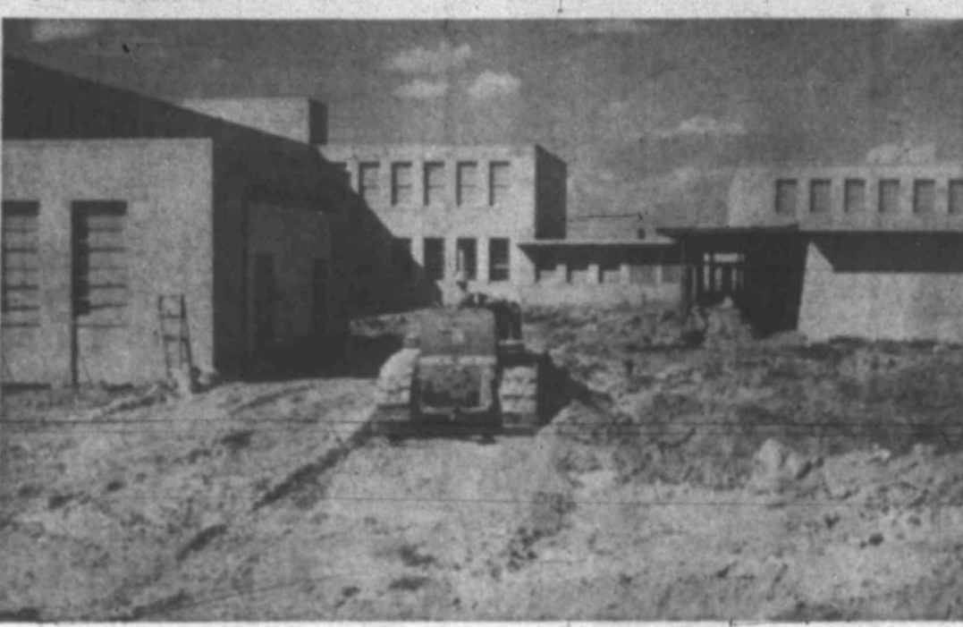
School Construction Progresses
