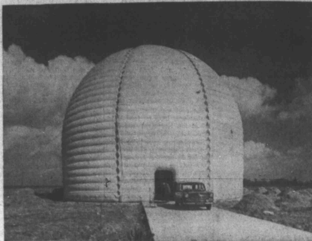
SPACE SYSTEM LINK —This radome is an incongruous sight in a rural setting at Christchurch, England. It houses an earth station to be used to send and receive military communications under an Anglo-American defense system of space satellites.
